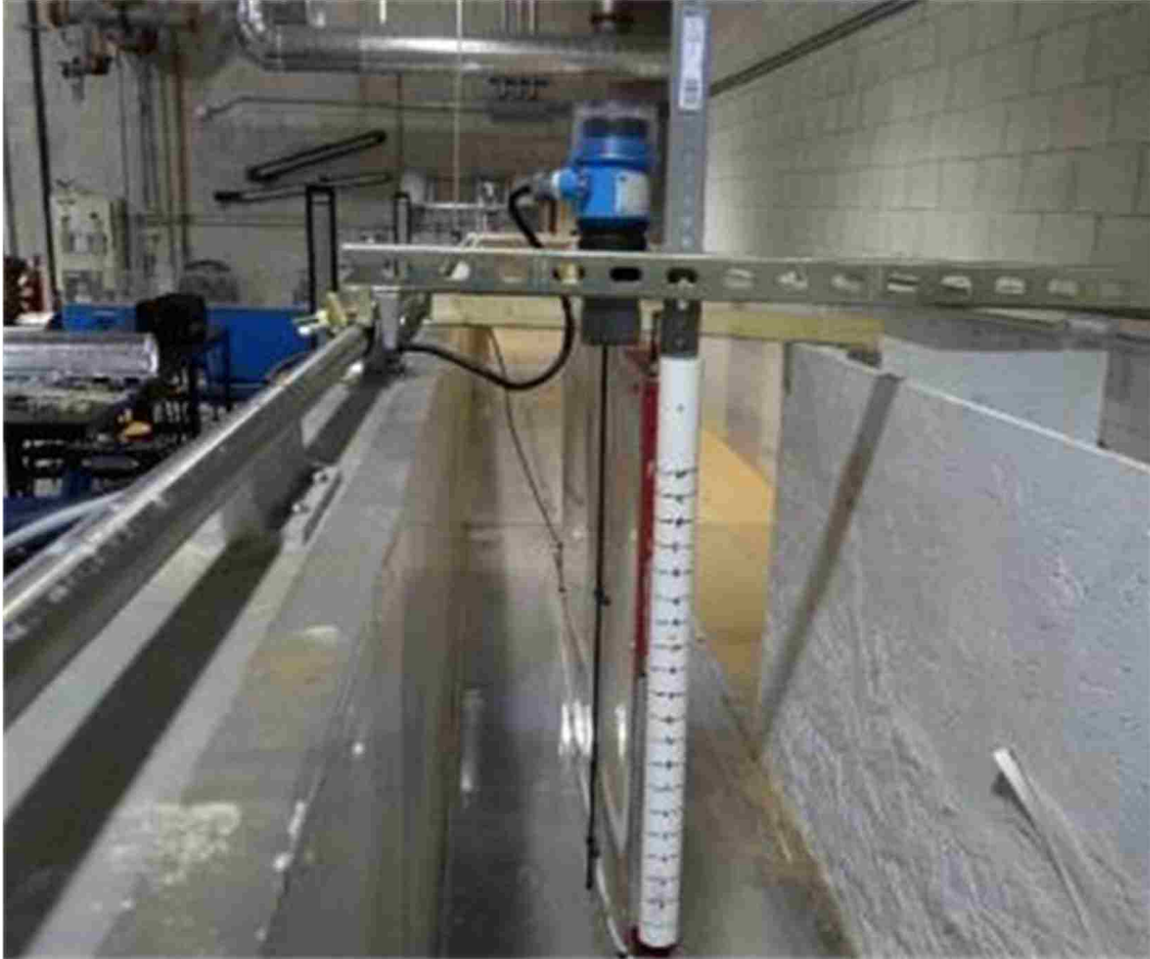
Figure 17. Level meter location, UNLV flume
